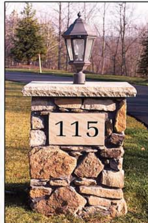
Indian Creek Splitface, Quarry Top Rock Random with Amherst Buff Sandstone Cap & Address Block
