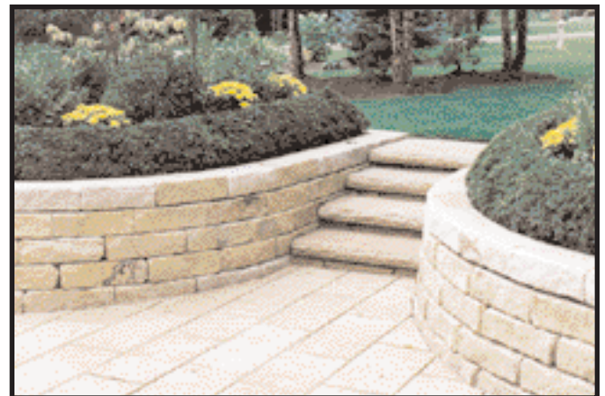
• Briar Hill Wall and Walkway with Custom Briar Hill Treads
